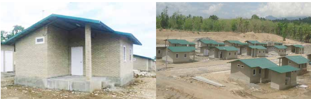
Construction progress of the infrastructure facilities for the support of Suai airport
