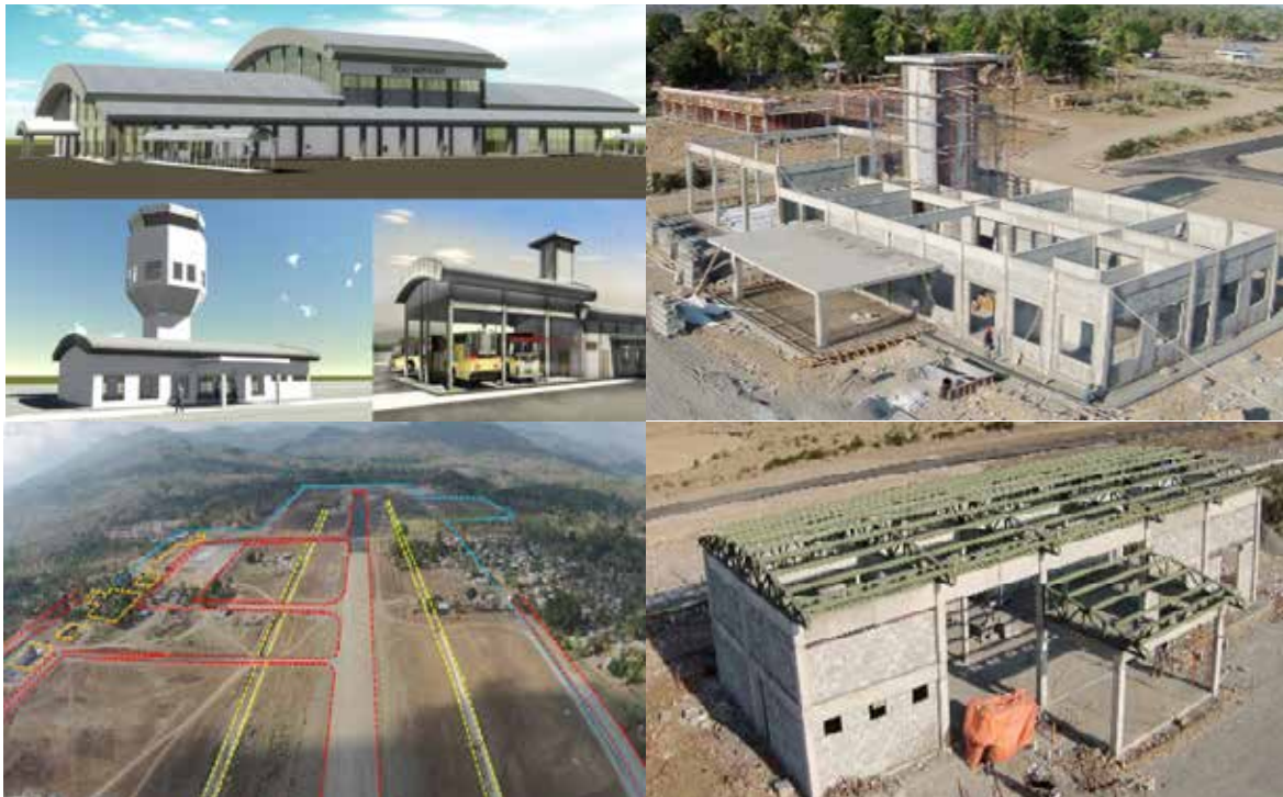
From top to bottom (left to right): Suai airport design; Suai airport construction progress; Runway total area.
