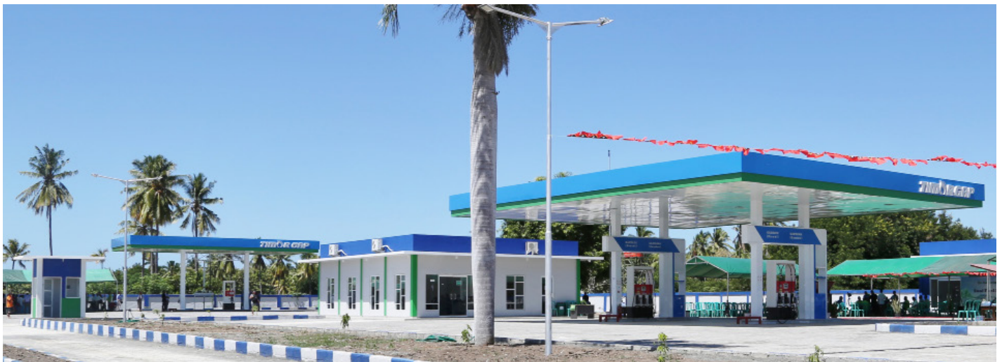
Suai Fuel Station
