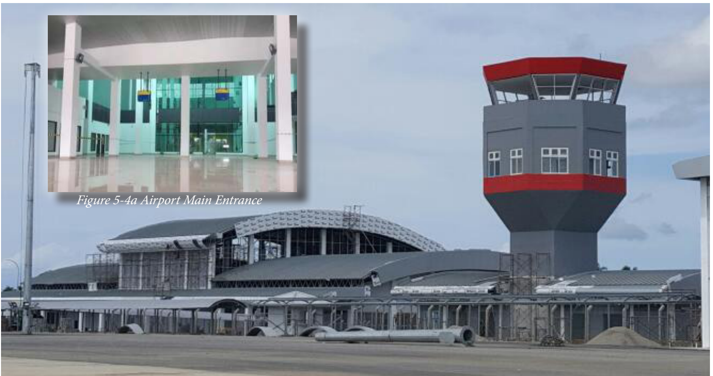
Figure 5-4b Suai Airport with Air Traffic Control Tower
