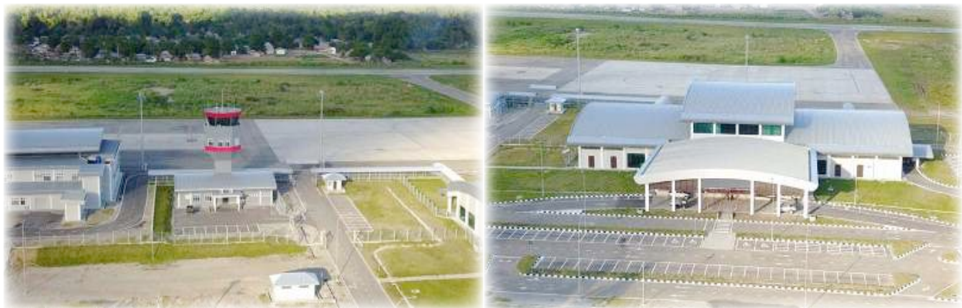
Figure 4-6: Air Traffic Control Tower (left); Airport new terminal building with facilities for security, customs and immigration (right)
