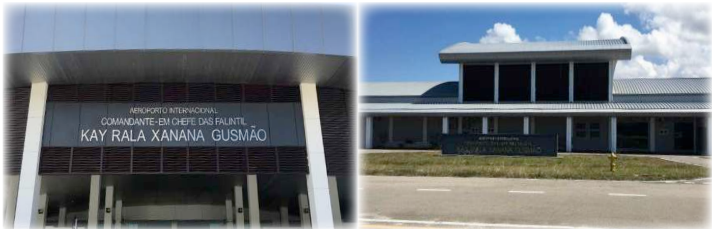
Figure 4-5: Main façade of the new terminal building
