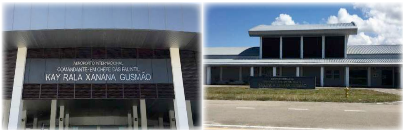
Figura 4-5: Fachada principal do novo terminal
