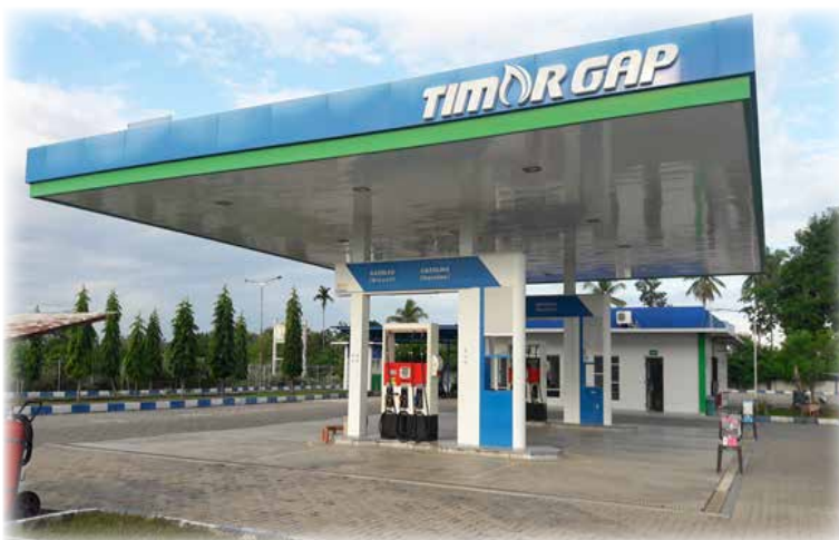
Figure 3-5: TIMOR GAP’s fuel station in Suai
