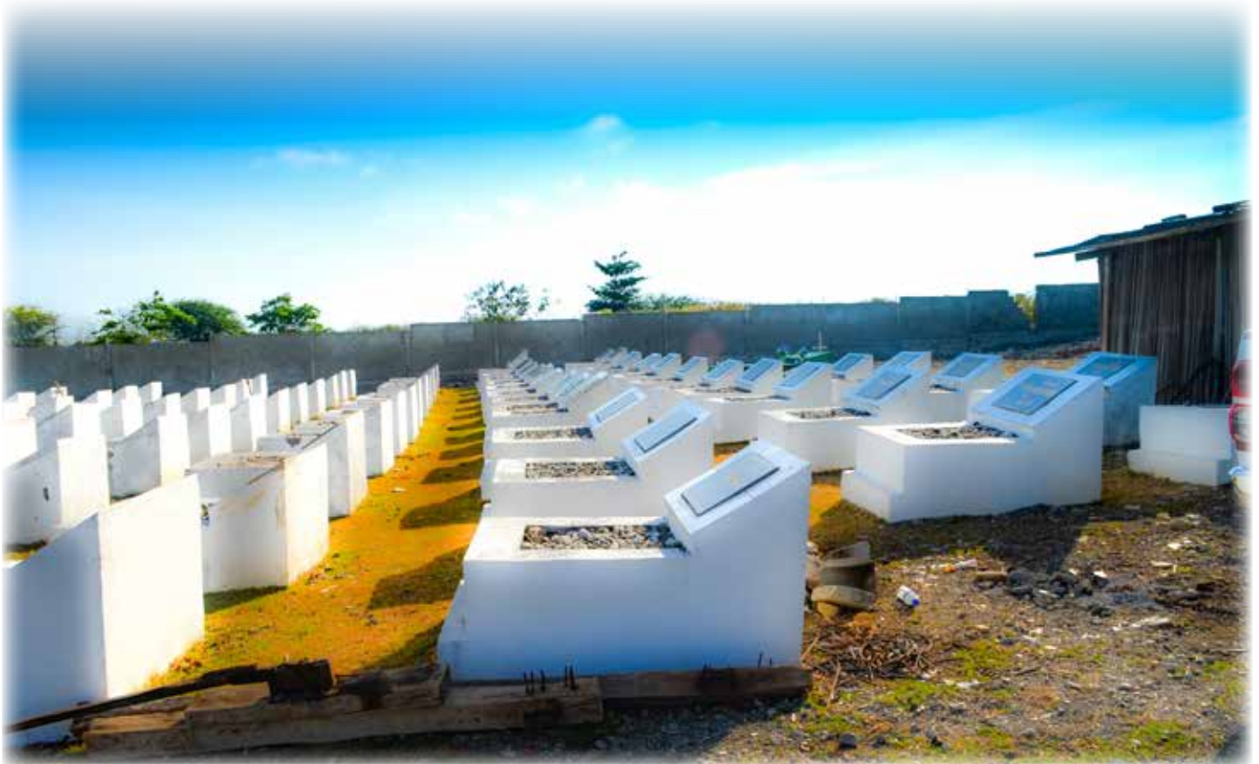
Figure 4-10: Permanent cemetery in Suai Airport (Phase I)
