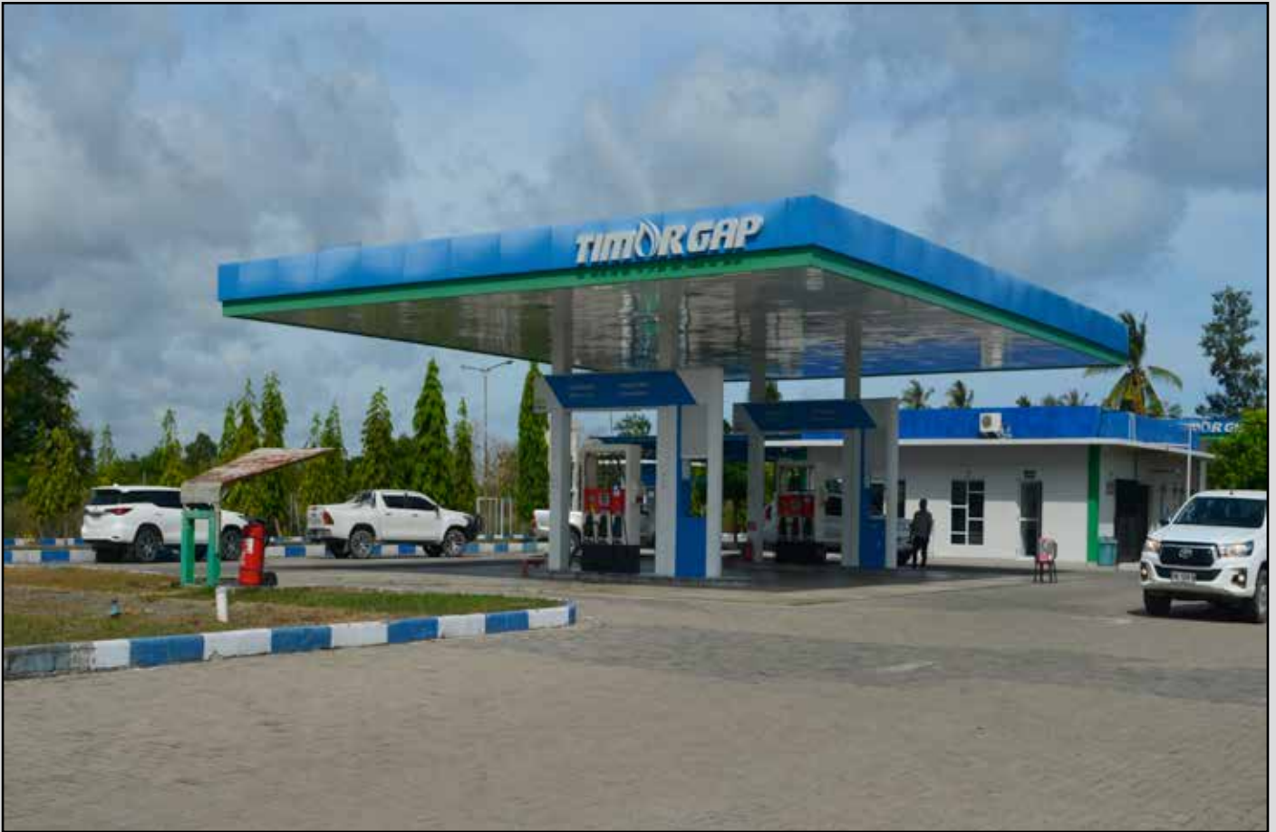
Figure 3-1: TIMOR GAP Retail Fuel Station in Suai
