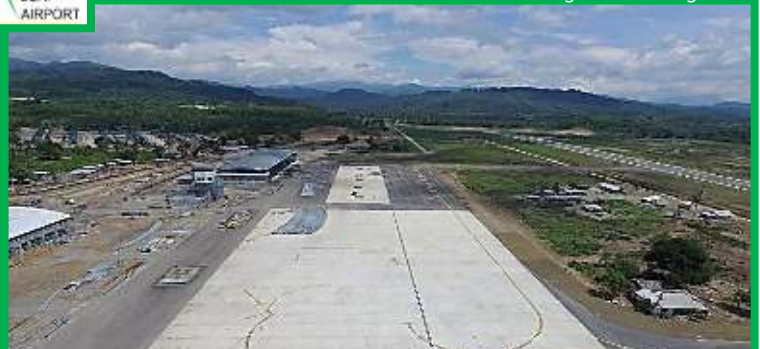
Ramp - Parking area
