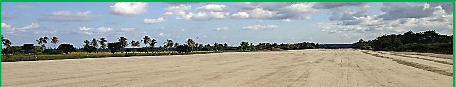
The highway will have four lanes (two in each direction) each 3.6m wide, with a total pavement width of about 26 m. Total length will be 155.7 km
