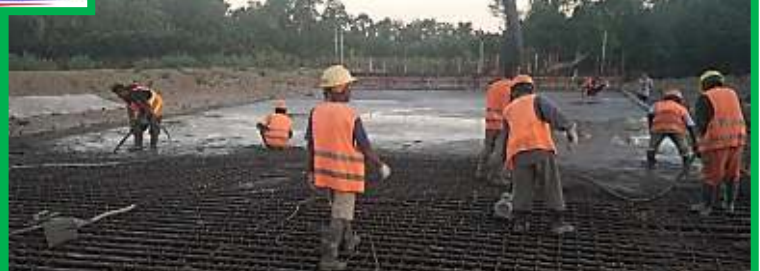
Walls & Top slab Concrete Pouring Ramp - Parking area
