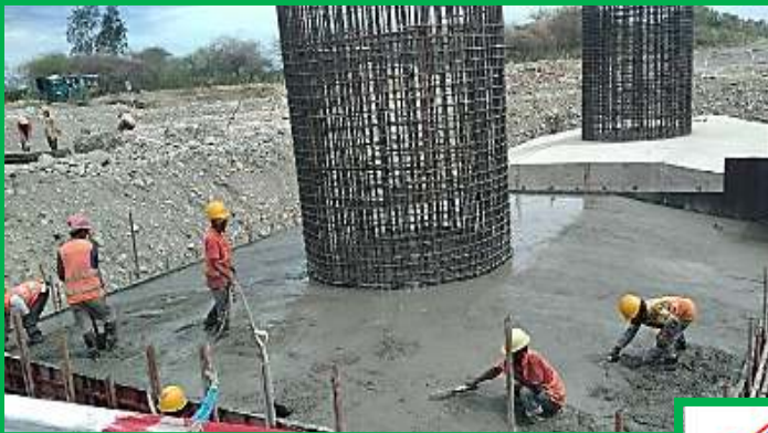
Mola Bridge Column of Pier
