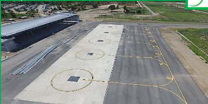
Parking area and Hangar for Helicopters
