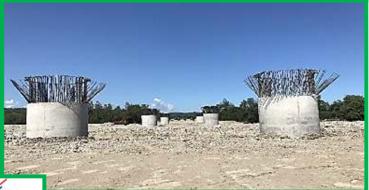
Mola Bridge Column of Pier
