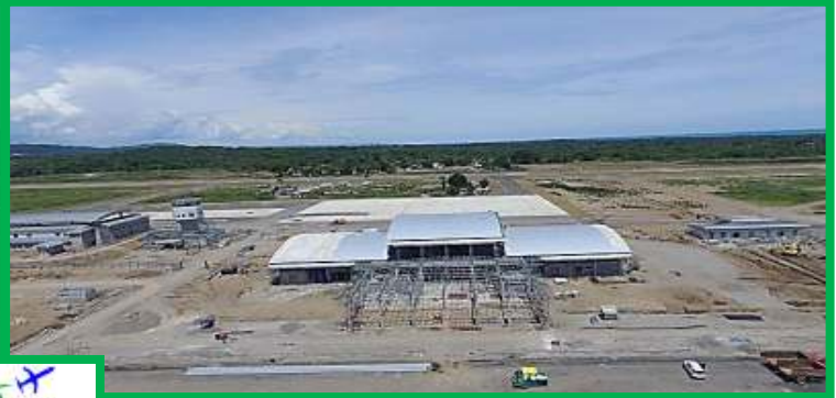
Main Terminal Building and Parking Area
