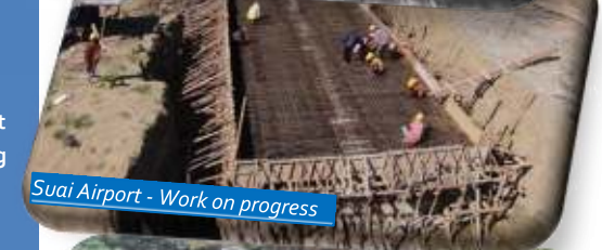
Airport area under construction
