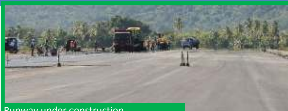
Runway under construction
