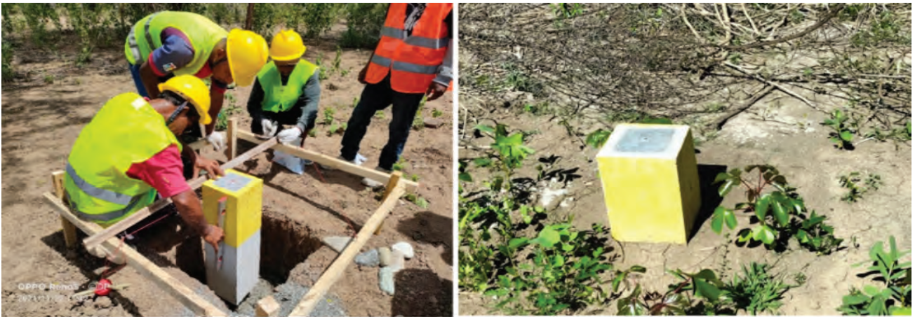
Figure 4-8: SSB benchmark progress installation
