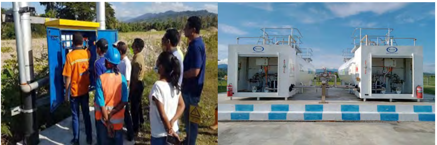
Figure 3-13: Inspection to the low voltage line (left); Fuel tanks (right)
