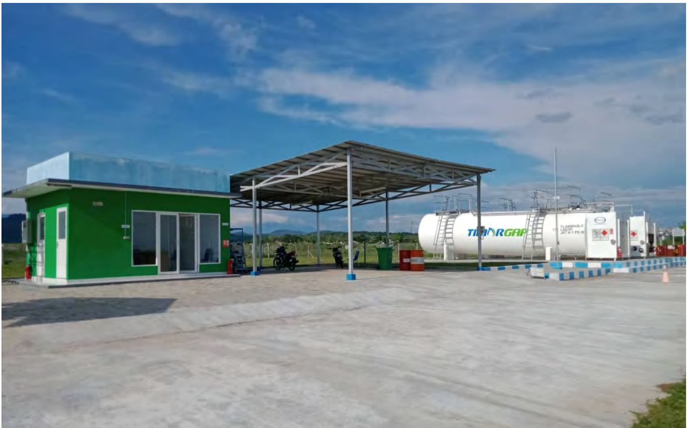
Figure 3-12: TIMOR GAP Aviation Fuel Facility in Suai
