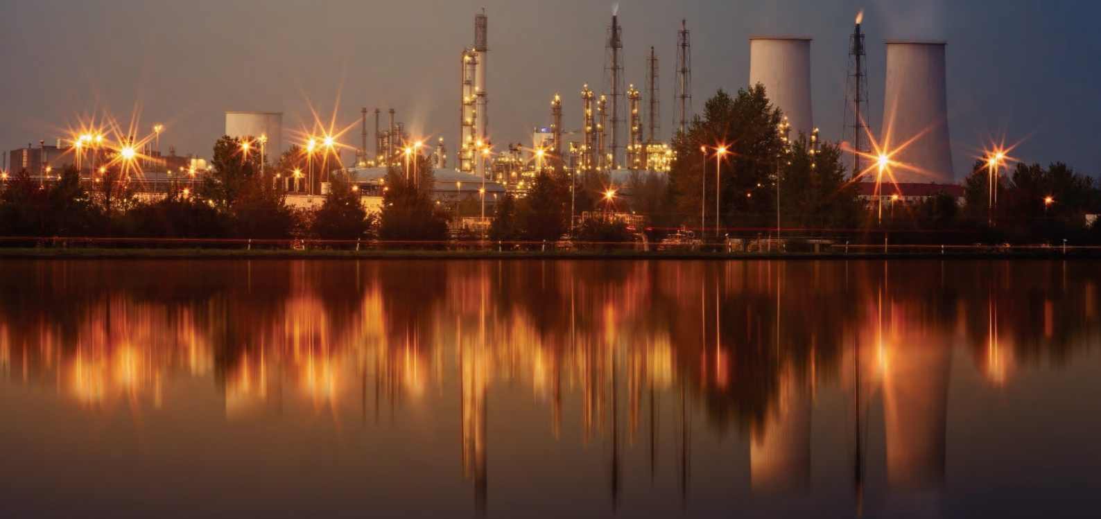
Figure 4-13: Typical Refinery & Petrochemical Plant
